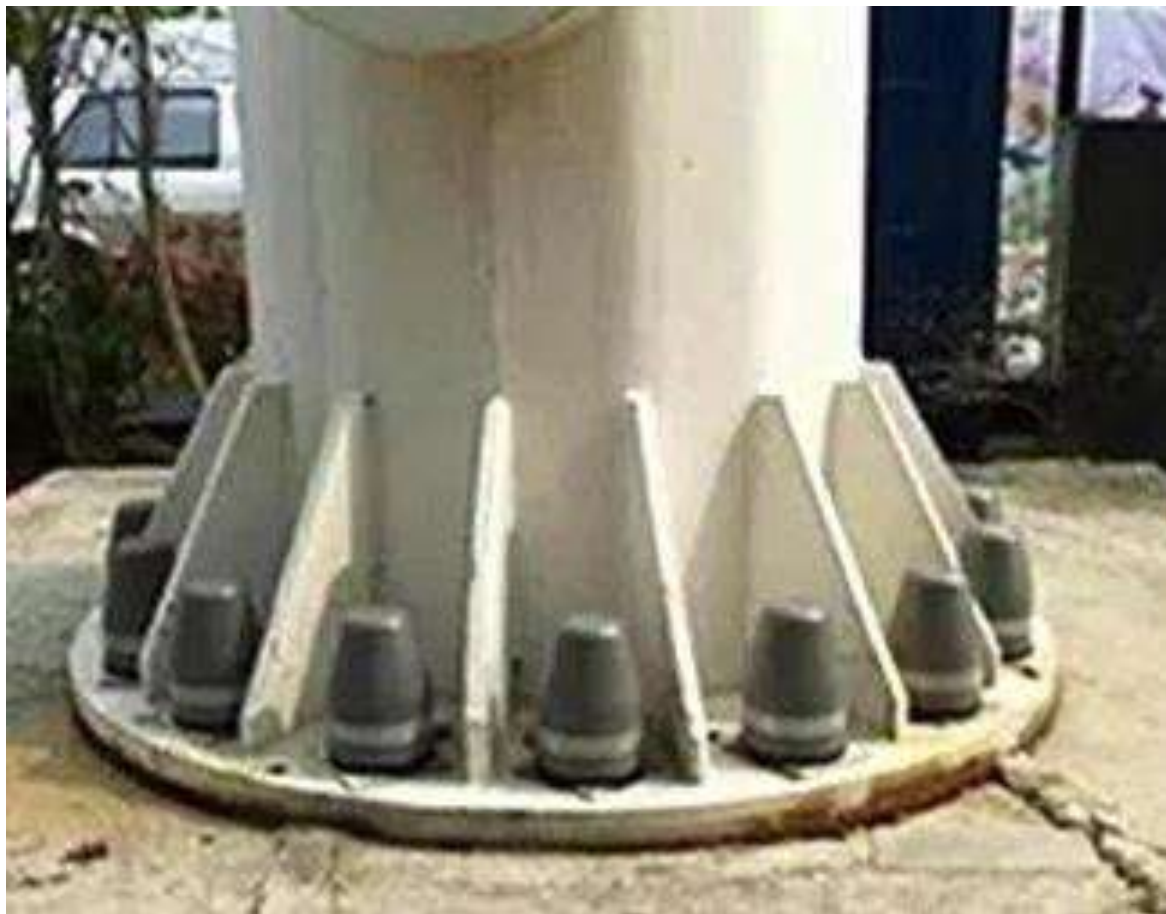
Fig: Typical footing including base plate and anchor bolt
